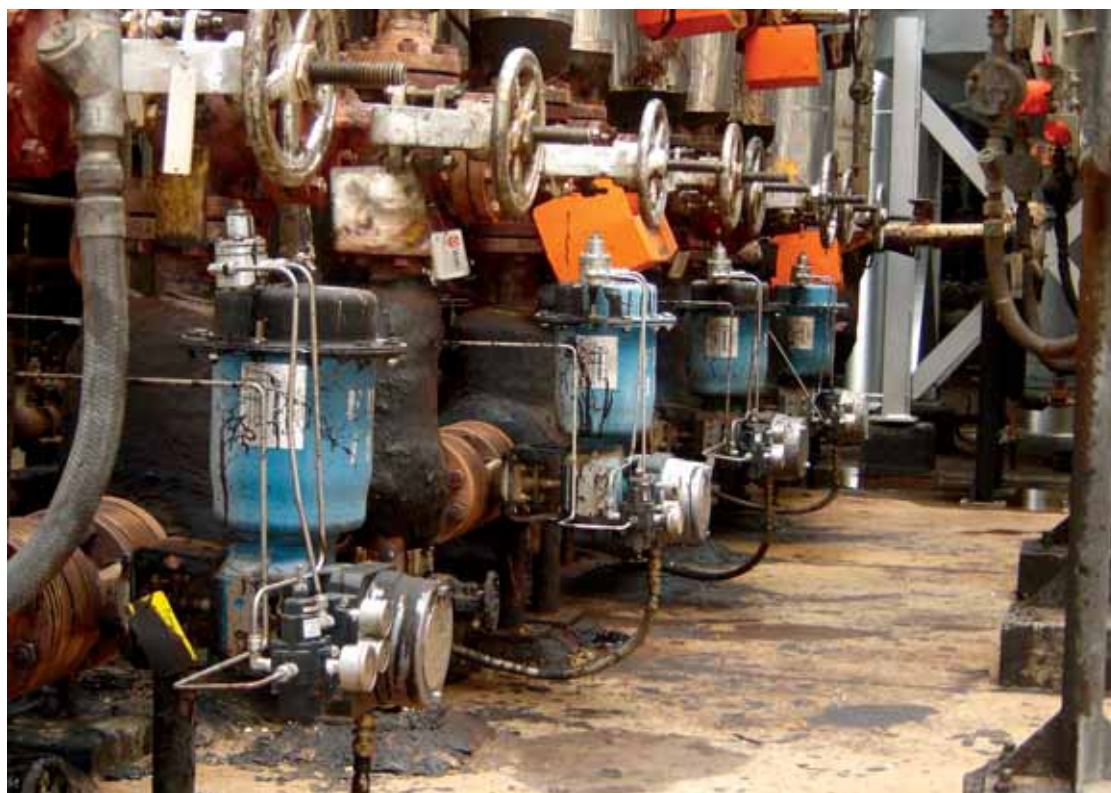
Finetrol control valve is the preferred solution for heater-pass applications at Petrobras.
